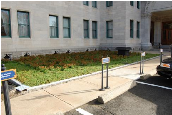
Figure 3.13 – Bioretention retrofit.
