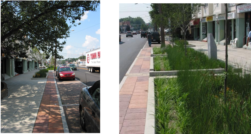
Figure 3.12 – Permeable pavement (left photograph) and rain garden/bioretention (right photograph) retrofits along North Main Street in Bridgeport, CT.
