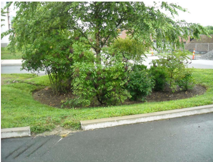
Figure 4.26 – Bioretention at University of Connecticut Storrs Campus –Mansfield. Source: Connecticut Department of Environmental Protection.
